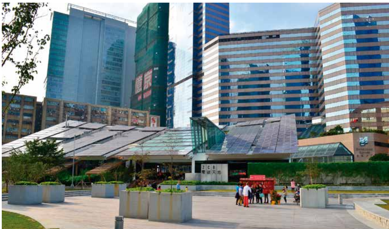
Zero Carbon Building – Hong Kong
